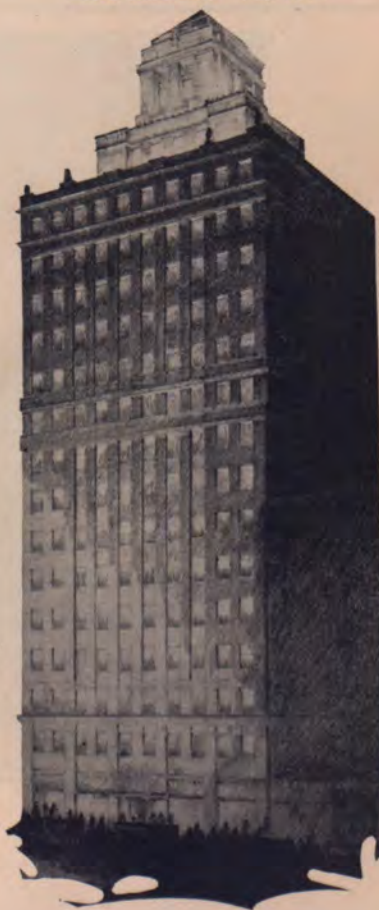
THOMPSON BUILDING After December 1st, 1929
