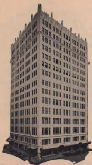
T. A. Hunt, Building Manager, Telephone 4-1616
