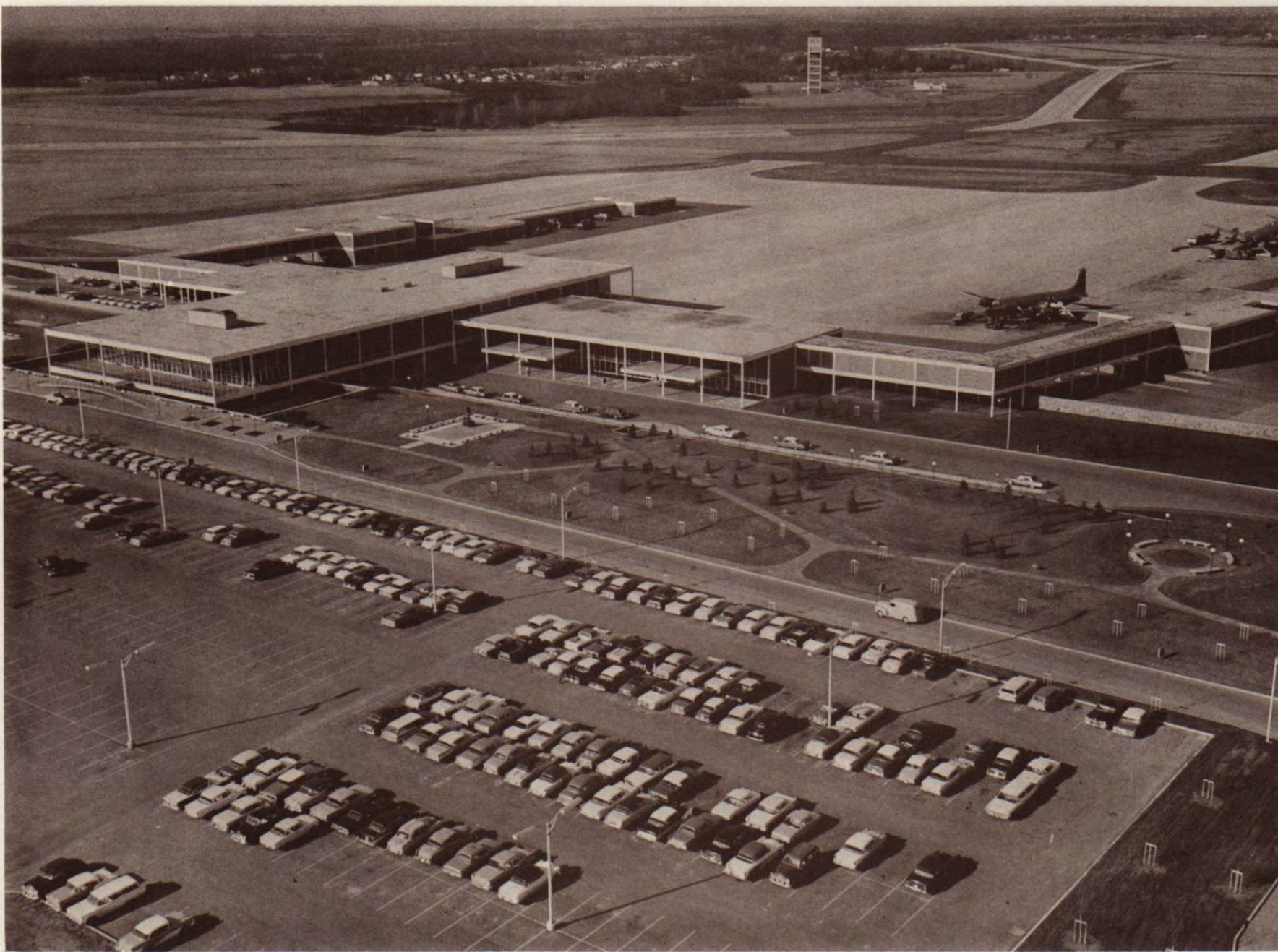
TULSA MUNICIPAL AIRPORT TERMINAL BUILDING Tulsa, Oklahoma Murray-Jones-Murray, Architects
