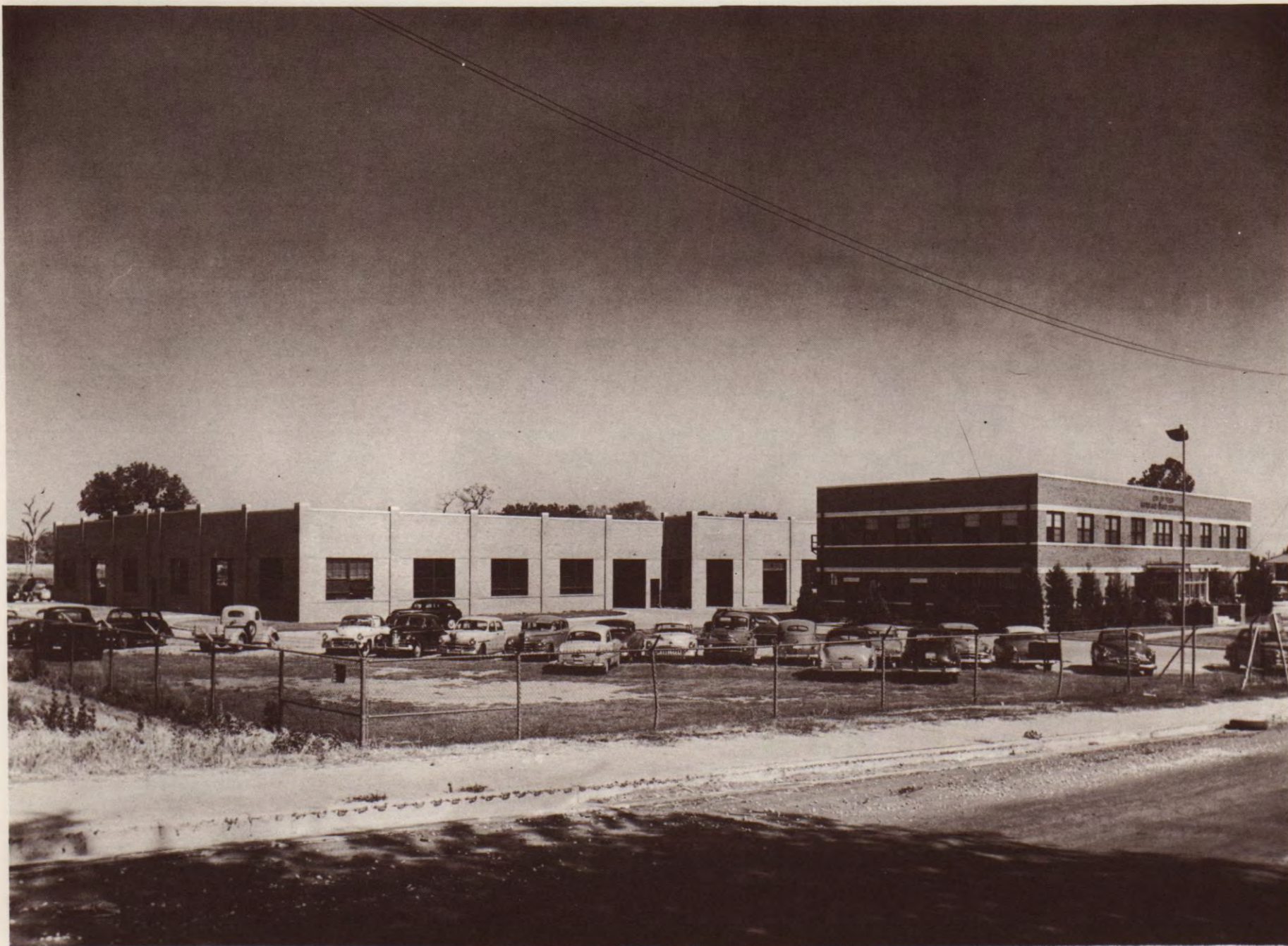
WAREHOUSE BUILDING, CITY OF TULSA
