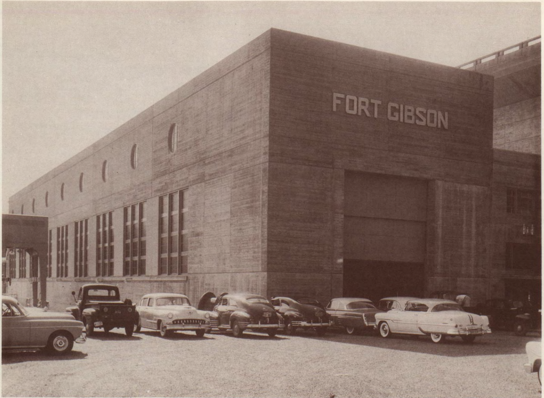
FORT GIBSON HYDROELECTRIC POWERHOUSE Grand River, Oklahoma Corps of Engineers, U. S. Army
