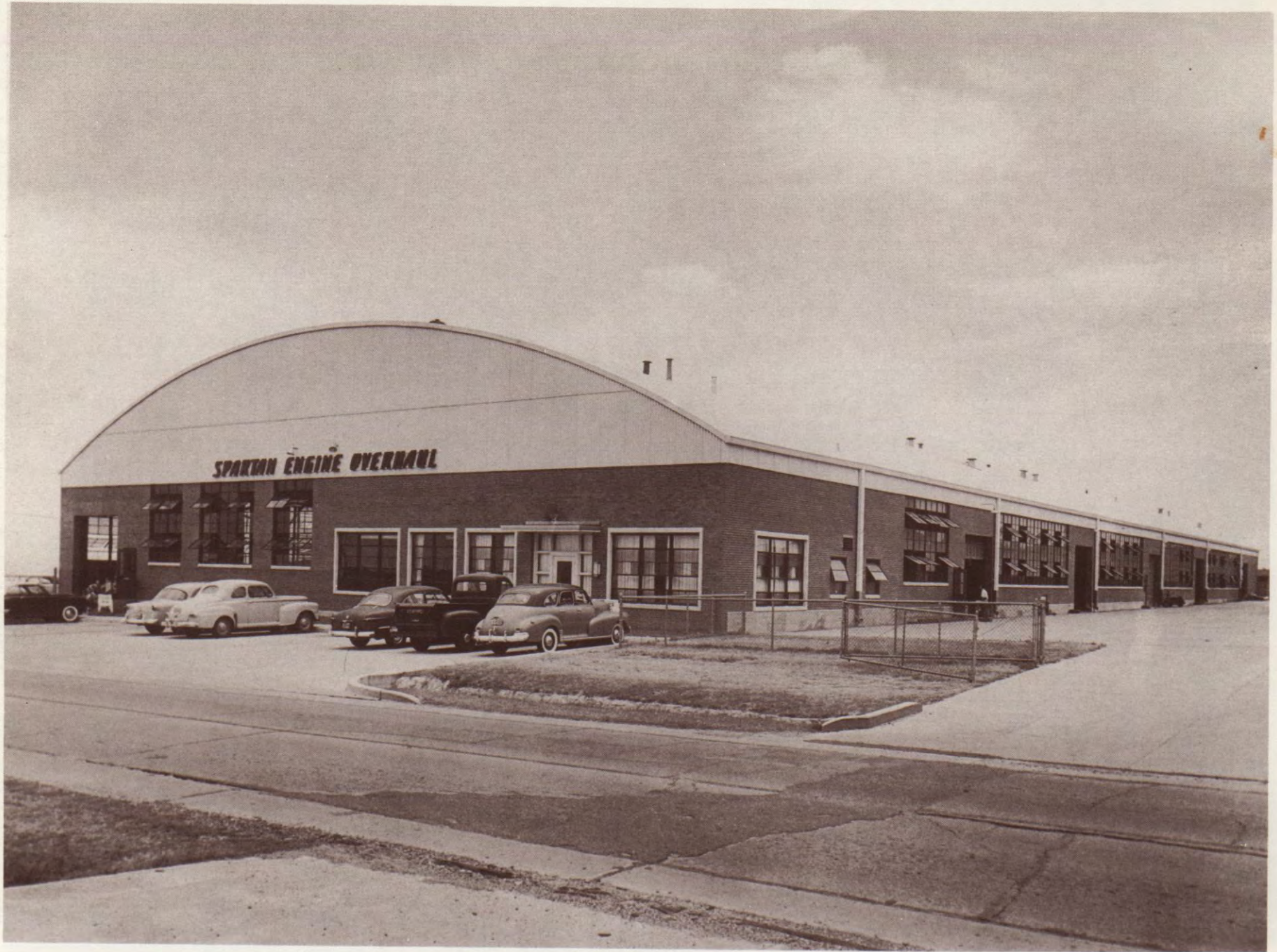
AERO REPAIR BUILDING, SPARTAN SCHOOL OF AERONAUTICS Tulsa, Oklahoma Black & West, Architects
