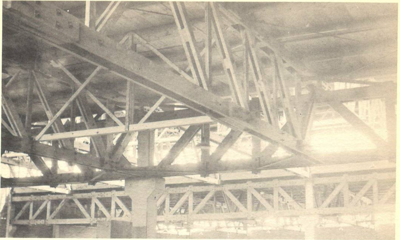
WOOD TRUSS CONSTRUCTION SUBSTITUTES FOR STEEL WHEN STEEL NOT AVAILABLE
