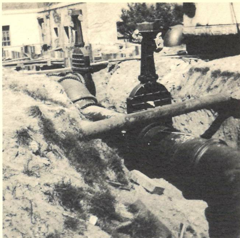
TYPICAL CIRCULATING WATER PIPING
