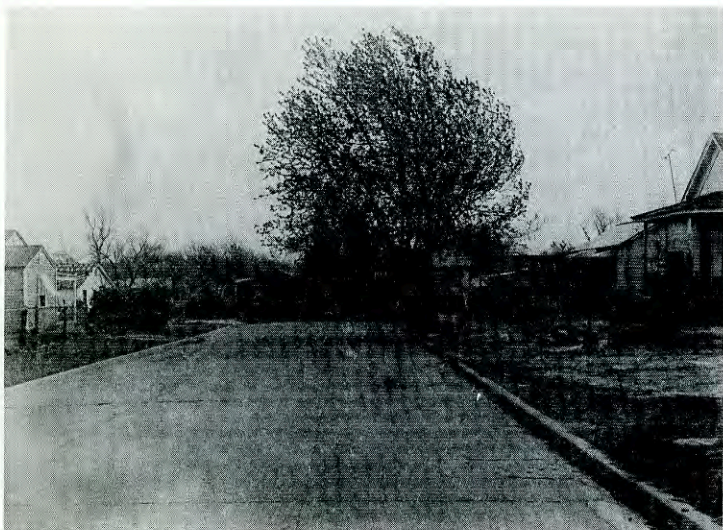
600 Block E. Reading, new paving but sub-standard housing and lack of cul-de-sac makes this an undesirable location.
