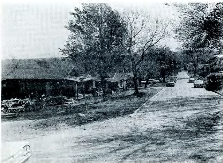
"Row" housing at No. Frankfort and E. Jasper Streets, steep hill and lack of paving on E. Jasper makes this an undesirable location.
