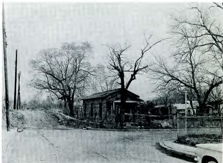
703 E. Reading, sub-standard housing in neighborhood of good homes and new paving, street improvement and removal of this type of housing would make this a valuable location.
