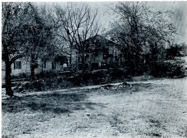
Extreme topography, lack of paving, and burned-out house decreases the value of this neighborhood at N. Frankfort and E. Jasper Streets.
