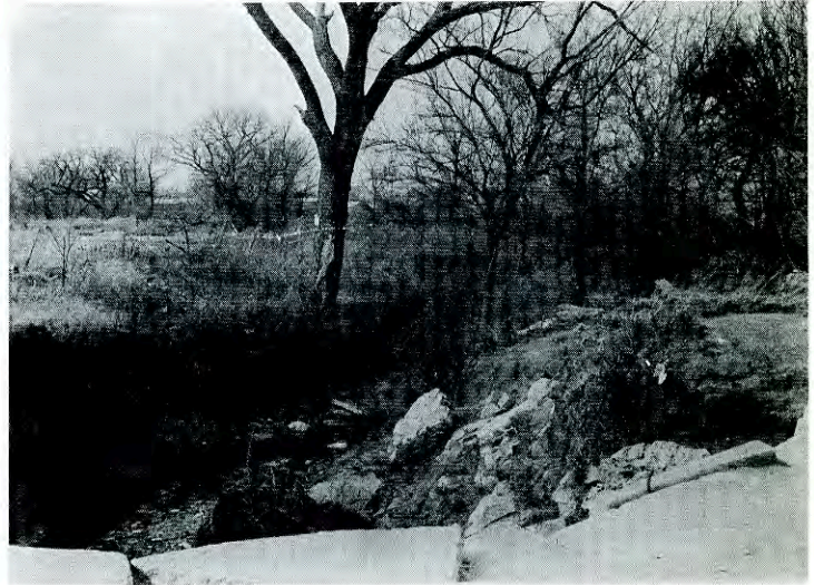
City park at 1700 Block E. Virgin end of large storm sewer project can be seen in foreground.
