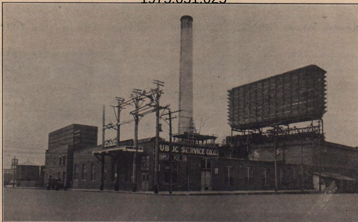
The old plant of the Public Service Company now being used as a sub-station and ice manufacturing.
