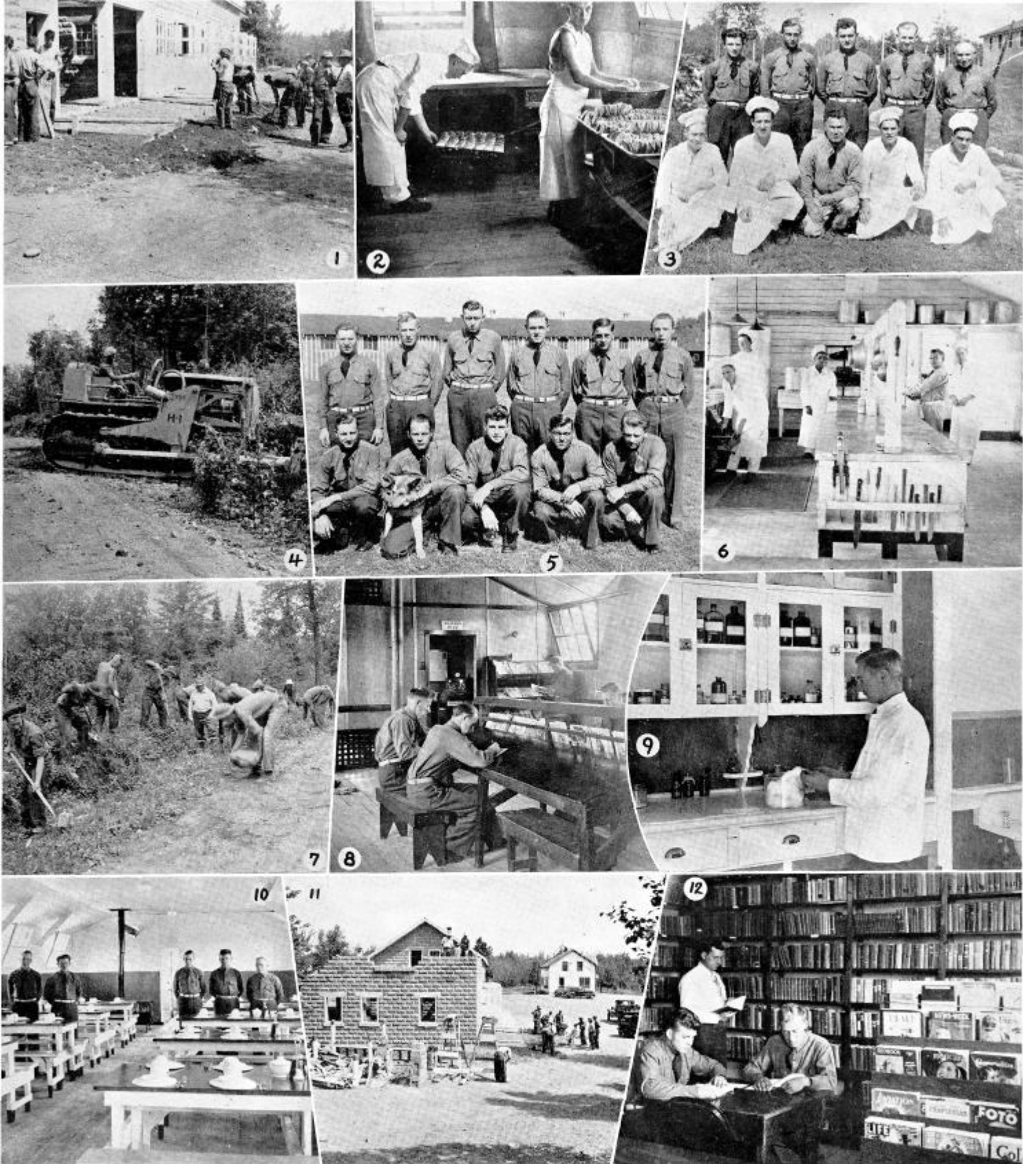
1. Finishing the front of the Ranger Station.
