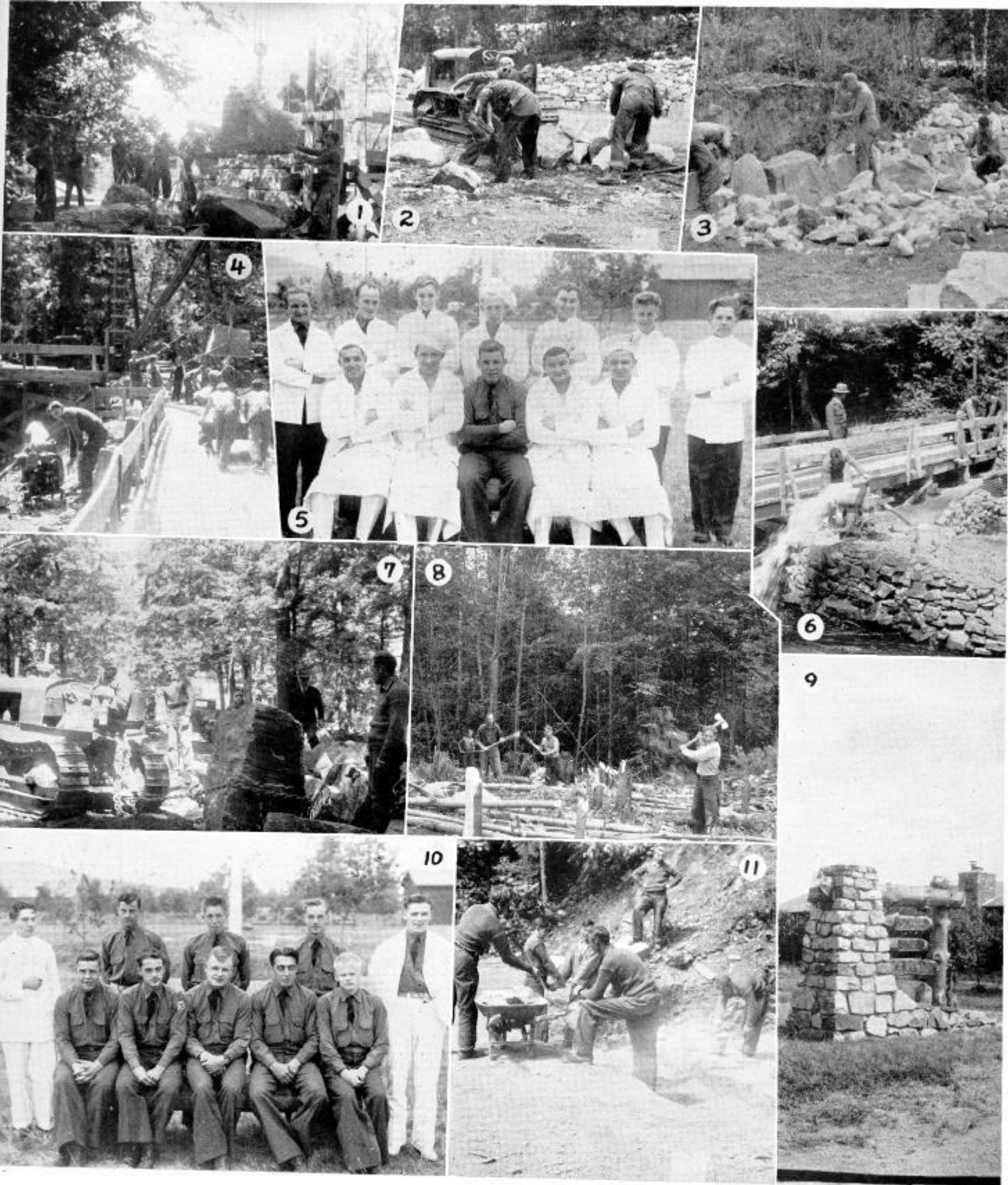
1. Erecting a stone pier.
