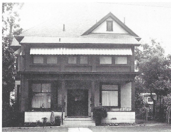
Barnes house – 1986 167 North Myrtle Avenue (Photograph by Richard Izbicki)
