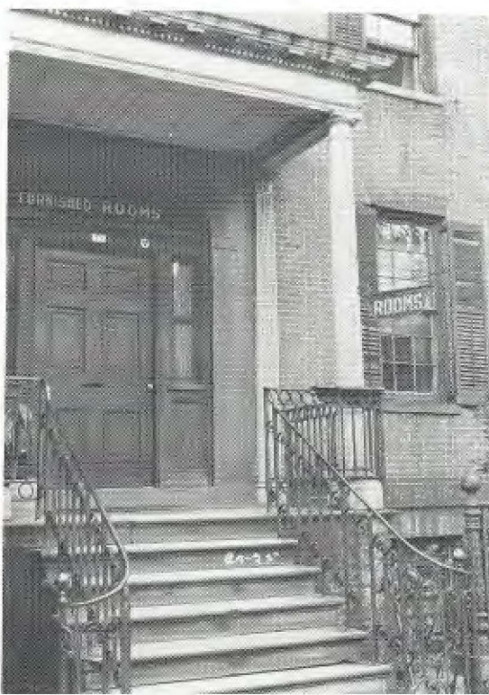
STURGES HOUSE was a rooming home in 1936, years before Historic Savannah preserved it for later restoration.
