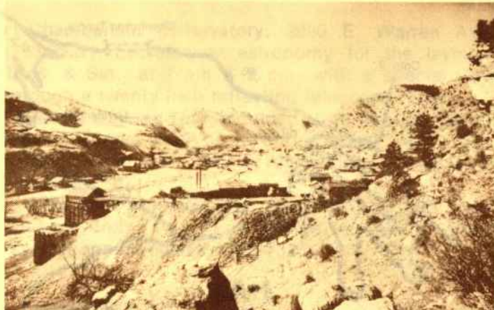
BOOMING IDAHO SPRINGS, seat of major gold discovery in 1859, had a long and prosperous mining life. Here is the Newhouse (later Argo) mill and tunnel which pierced deep under the mountains for five miles to tap mines as far away as Central City. Open for tours.
