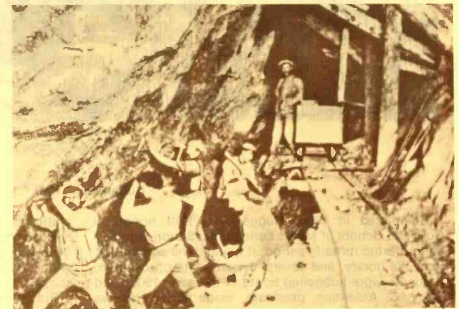
In the photo miners are drilling holes with double and single jacks.
