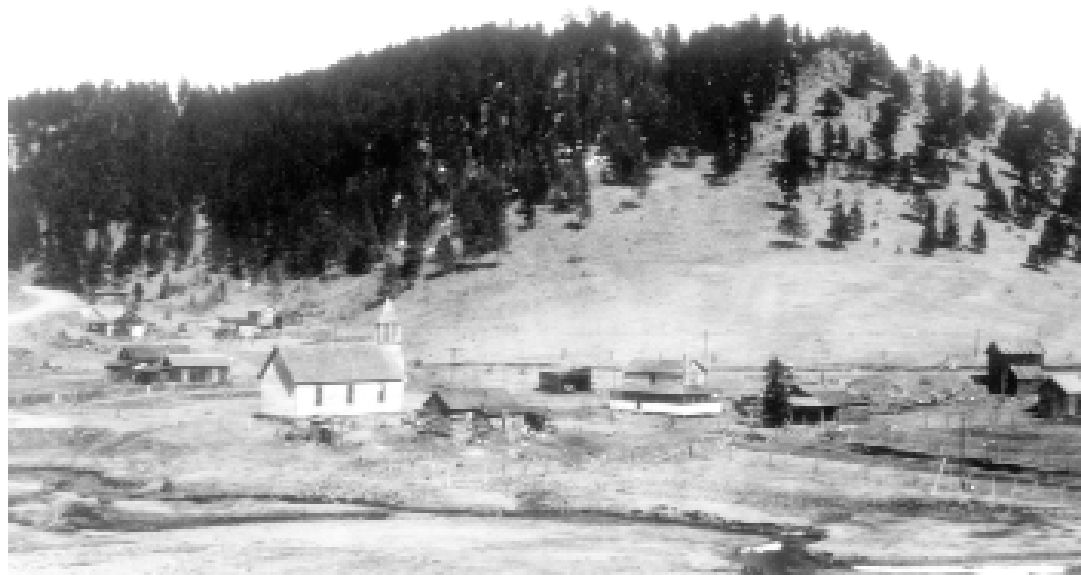
Shaffer's Crossing, early 1930s.
