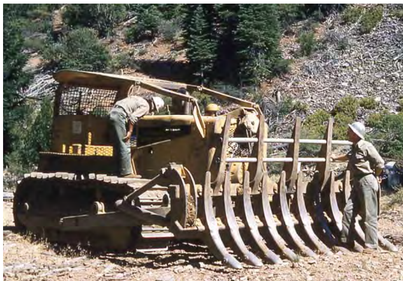
Brush rake used for site preparation
