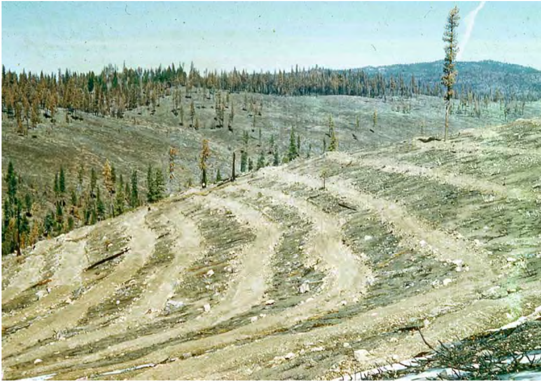
Terraces for erosion control and planting of the Donner Burn, 1961.
