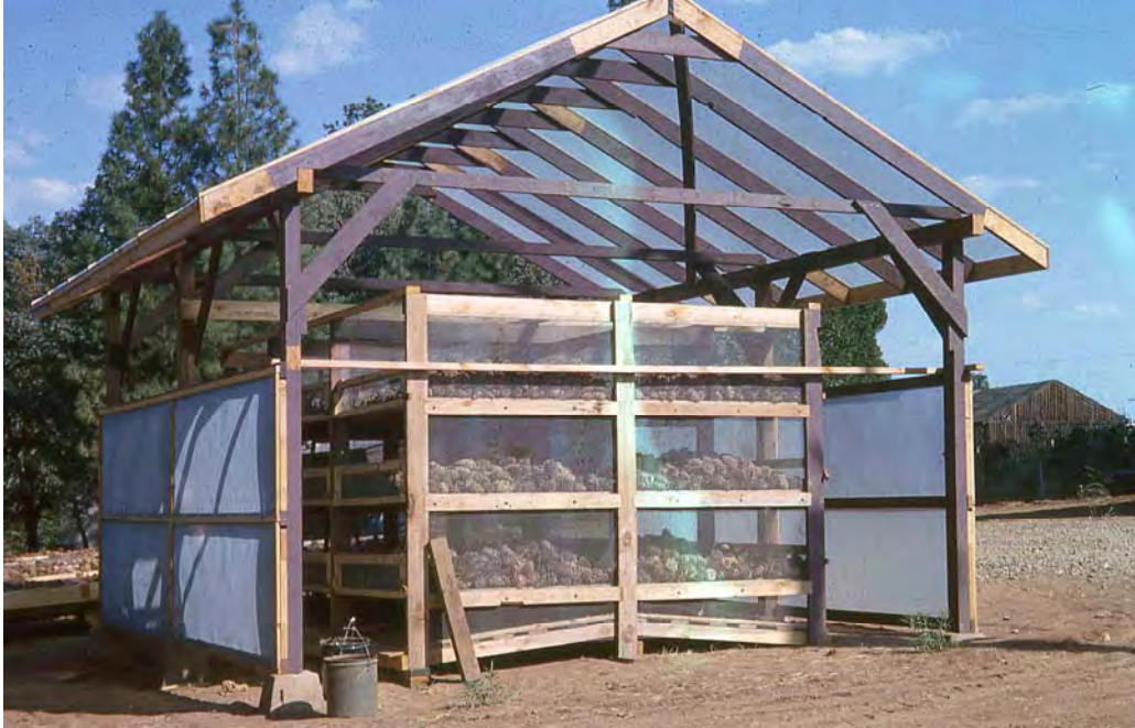
Cone drying shelter, Placerville Nursery, 1963.
