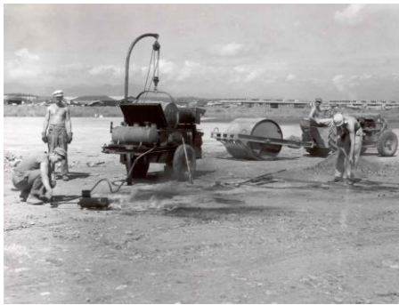
Figure 10 - Elements of the 872nd Airborne Engineer Battalion (Aviation) Refurbish portions of Atsugi Airfield at the end of WWII
