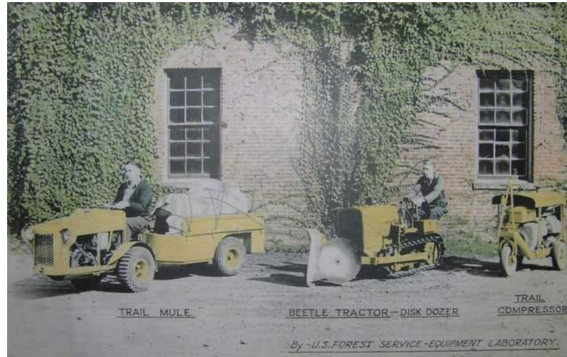
Figure 1 - Three pieces of trail maintenance equipment developed at the US Forest Service Equipment Development Laboratory during the 1940's - photo courtesy of the Oregon Historical Society
