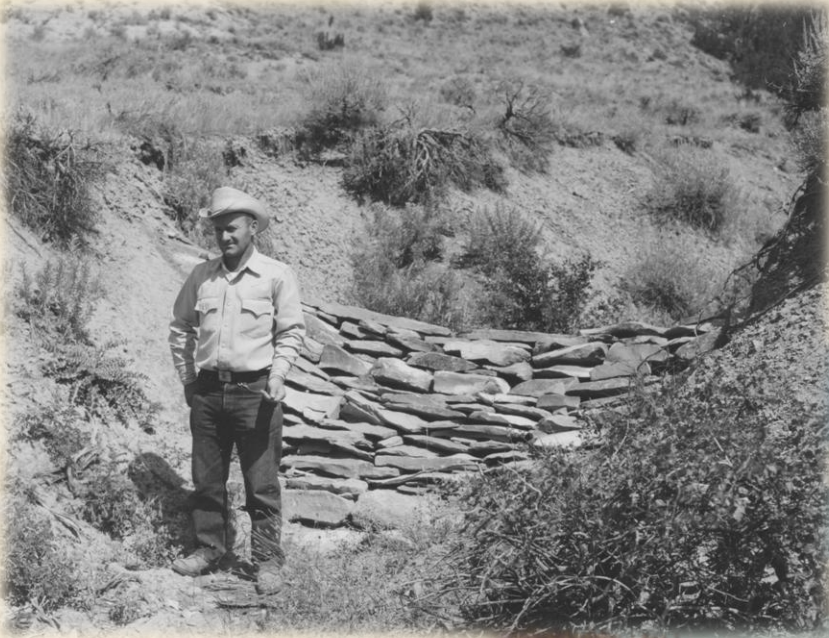
Shorty Creek rock check dam Ashland District- 1960
