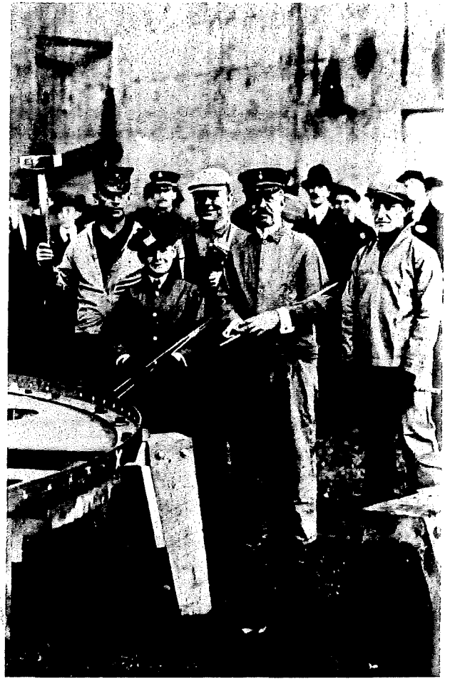
World War I Era—Submarine keel laying.
