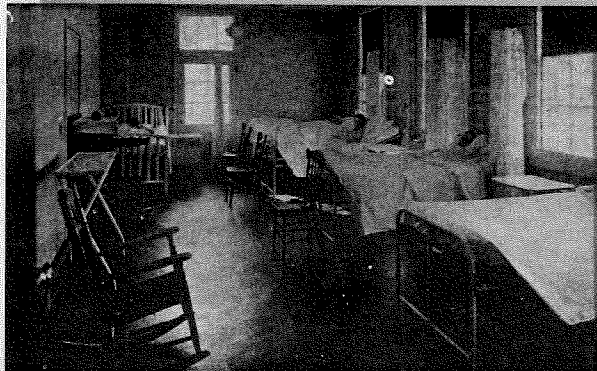
Ward, Cottage Hospital
