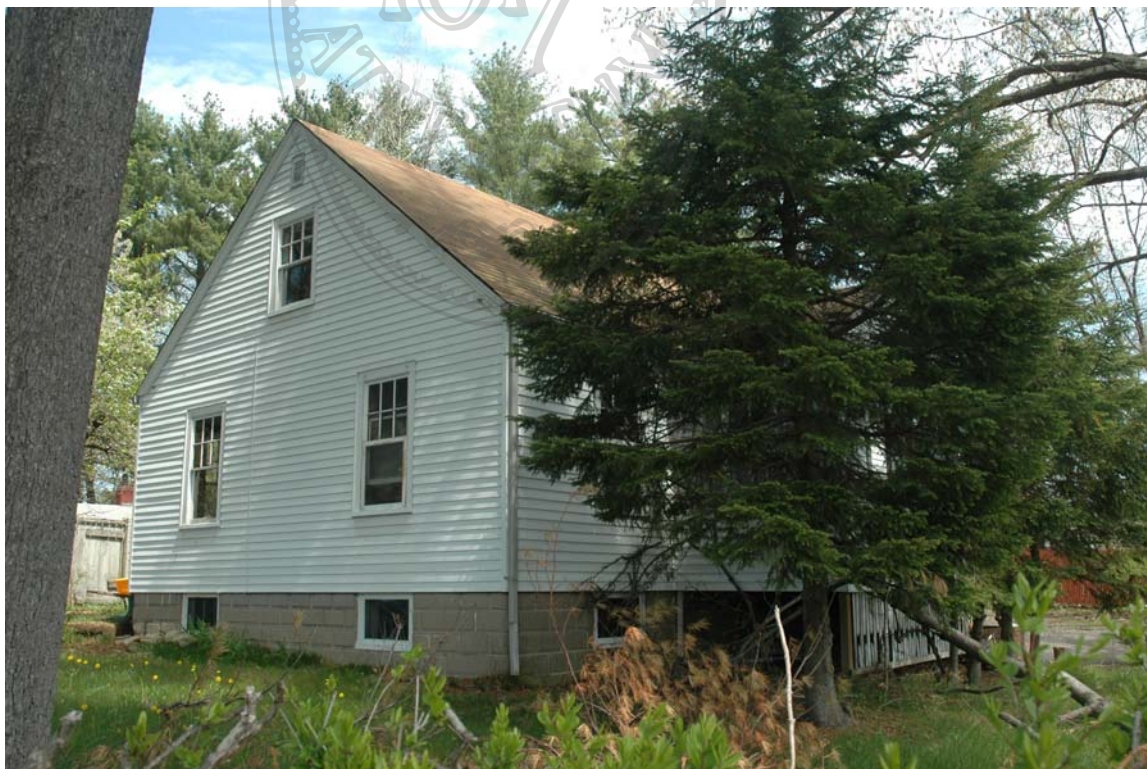
Photo 57) Route 1 Bypass, westerly side Direction: NW Digital File: ME-NH_0057
