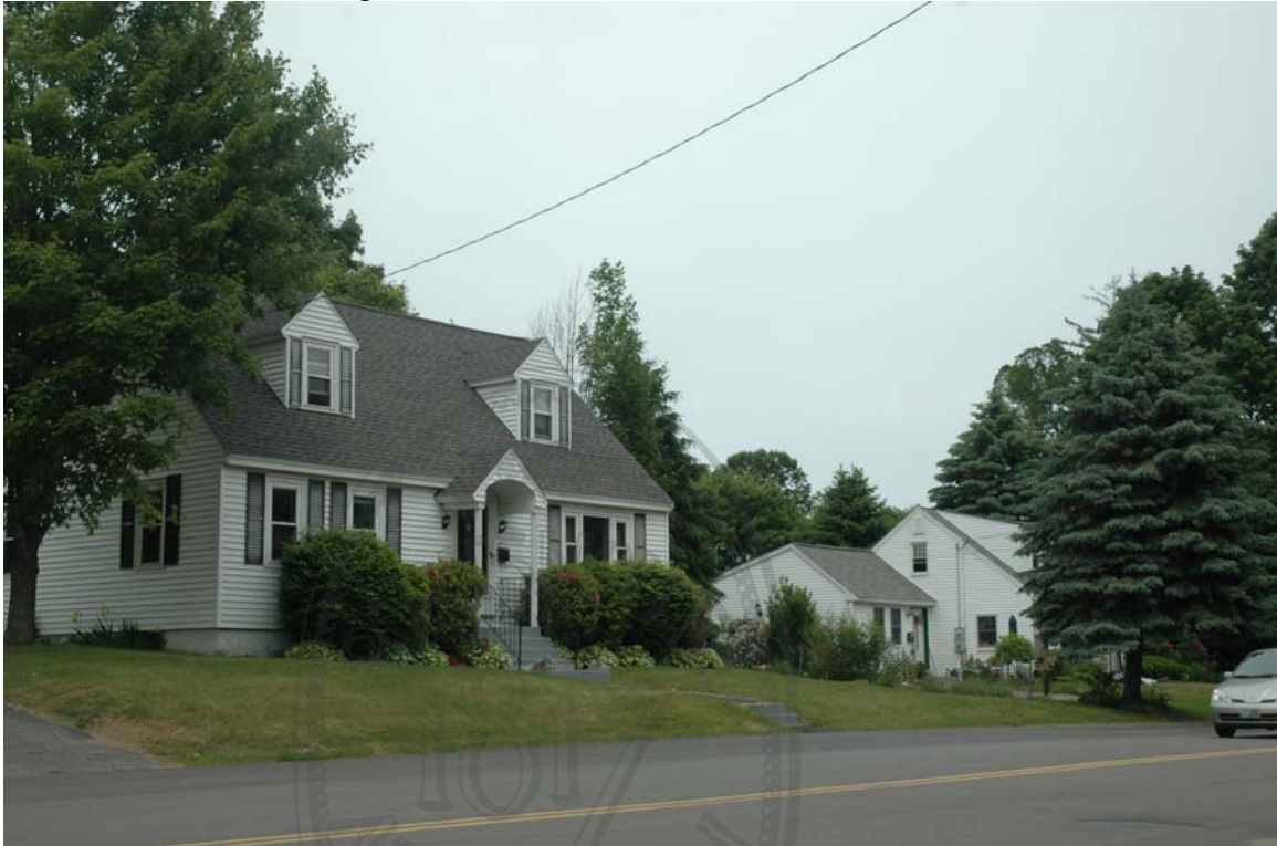
Photo 1) Maplewood Avenue at Central Avenue Direction: NE Digital File: ME-NH_0001
