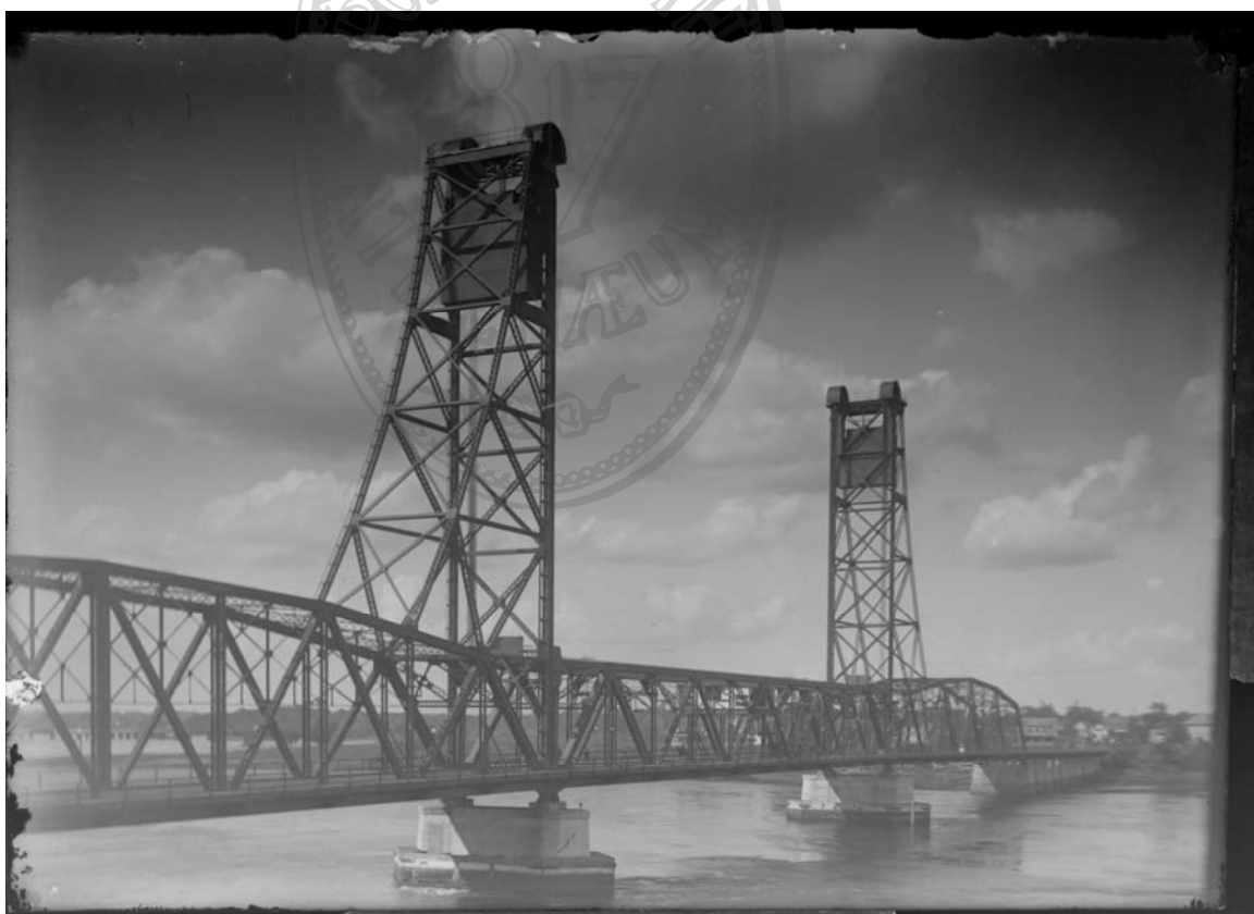
Historic Photo 79) Memorial Bridge, view from Navy Yard looking northwest towards Badger's Island. Photo J.F. Walker (courtesy of Kittery Historical Society, Image 0497136).
