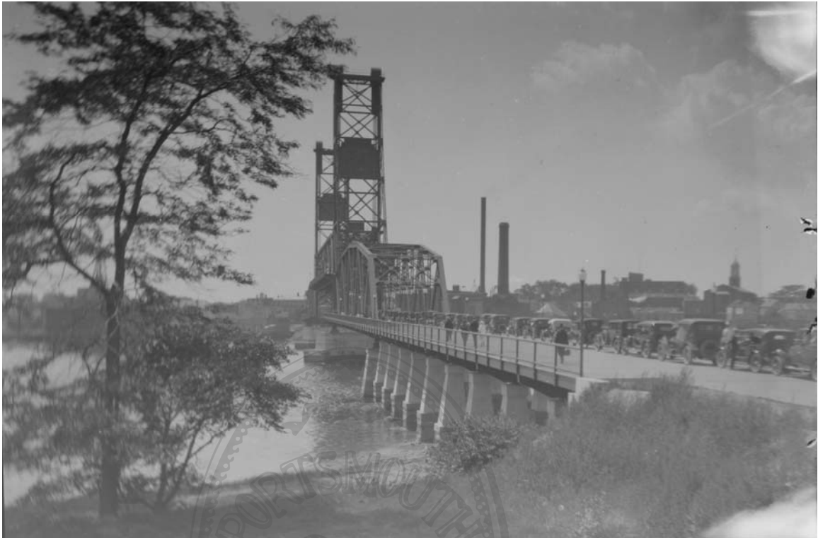
Historic Photo 80) Memorial Bridge, view from Badger's Island looking south towards Portsmouth showing pedestrian and vehicular traffic. Photo J.F. Walker (courtesy of Kittery Historical Society, Image 0500139).
