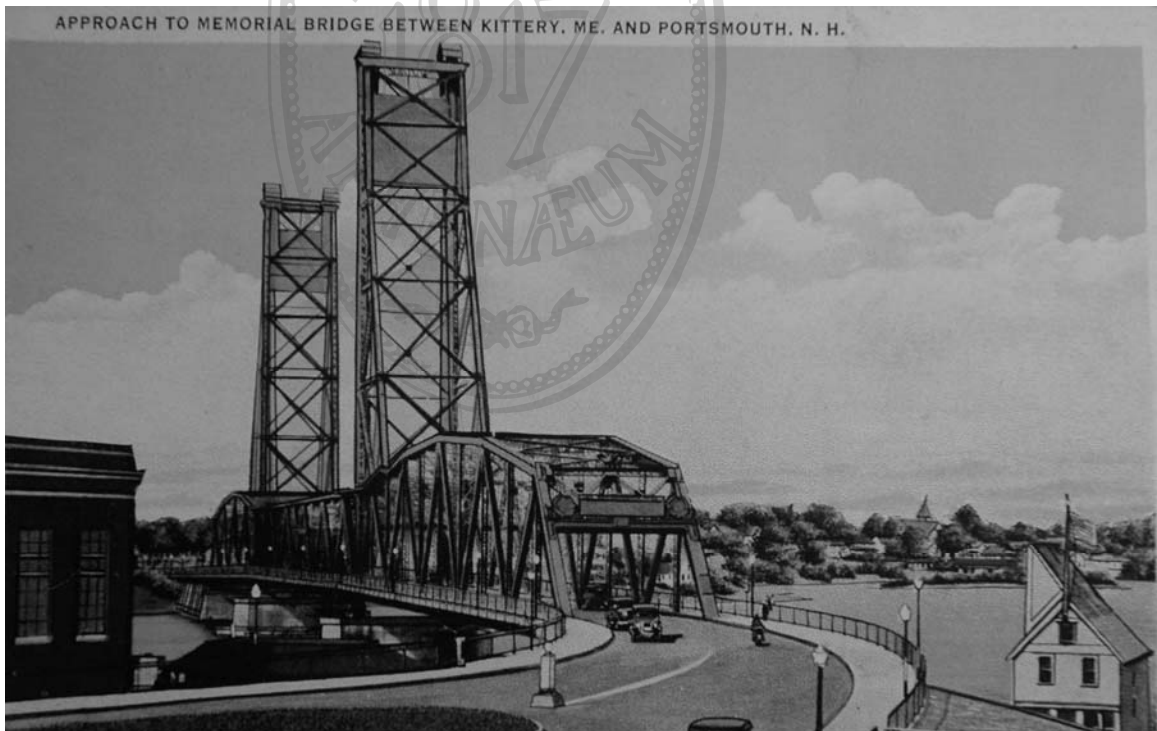
Historic Photo 83) Postcard. Memorial Bridge, approach from Portsmouth (Courtesy of Kittery Historical Society).
