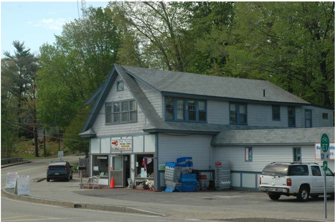
Photo 69) Dennett Road at Old Post Road, store Direction: SE Digital File: ME-NH_0069
