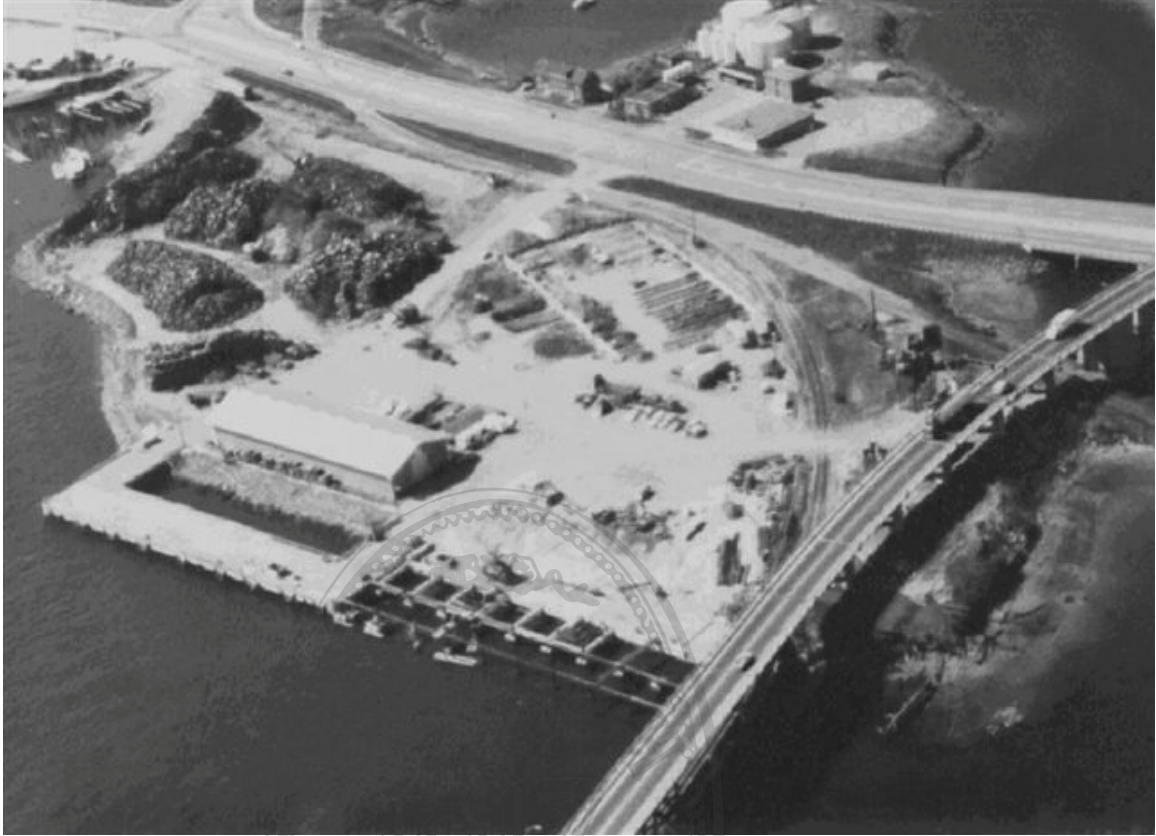
Historic Photo 18) Marine Terminal, before 1990s, before construction of wharf extension on northeast side of island (Courtesy of Captain Geno Marconi, Port Director, Portsmouth, Pease International Ports and Harbors).
