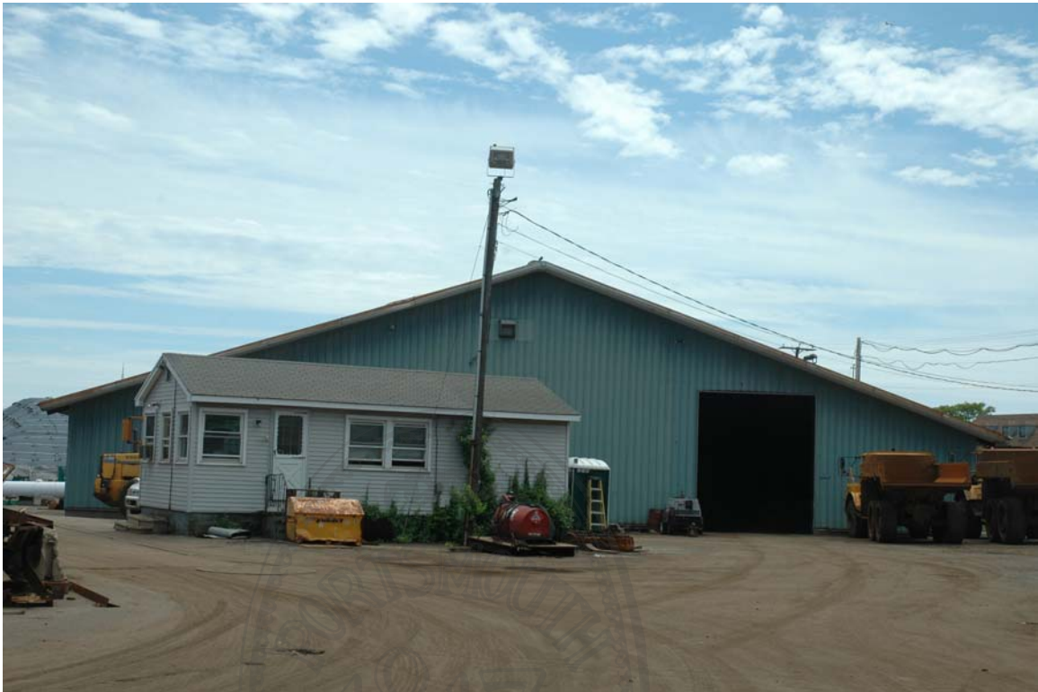
Photo 34) Port buildings, northwest elevations Direction: S Digital File: ME-NH_0034
