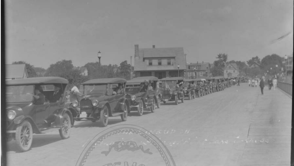
Historic Photo 67) Traffic waiting to cross Memorial Bridge. View looking north along Hunter Avenue across Badger Island's bridge to the mainland. The building in the middle ground is still extant. Photo J.F. Walker (courtesy of Kittery Historical Society, Image 0507146).
