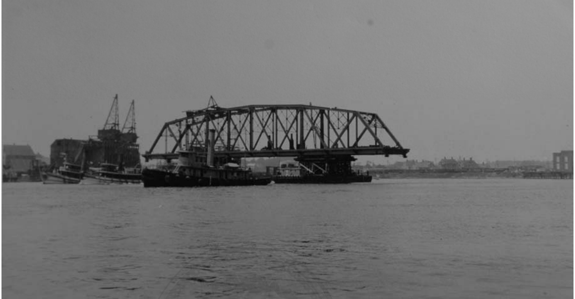
Historic Photo 86) Moving center span of Memorial Bridge into place (Courtesy of Kittery Historical Society).
