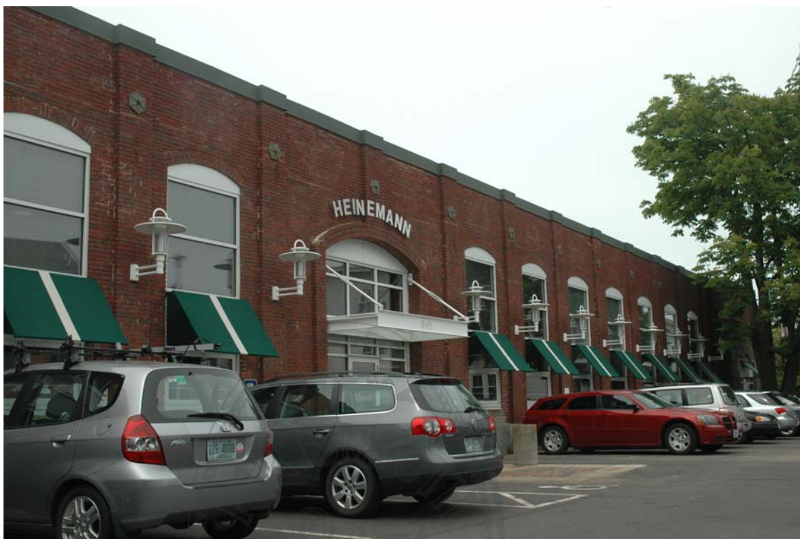
Photo 49) Hanover Street, northwest side, former Portsmouth Machine Company building Direction: N Digital File: ME-NH_0049
