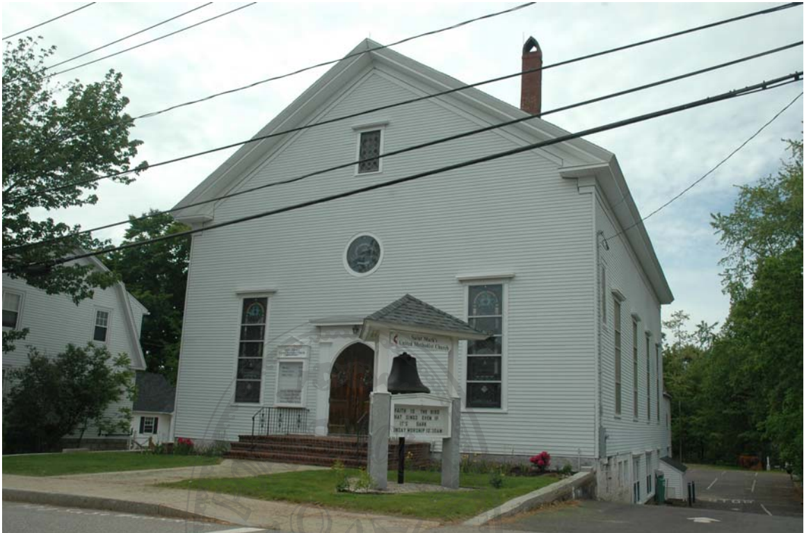
Photo 118) St. Mark's Church, Government Street, northerly side Direction: NW Digital File: ME-NH_0118
