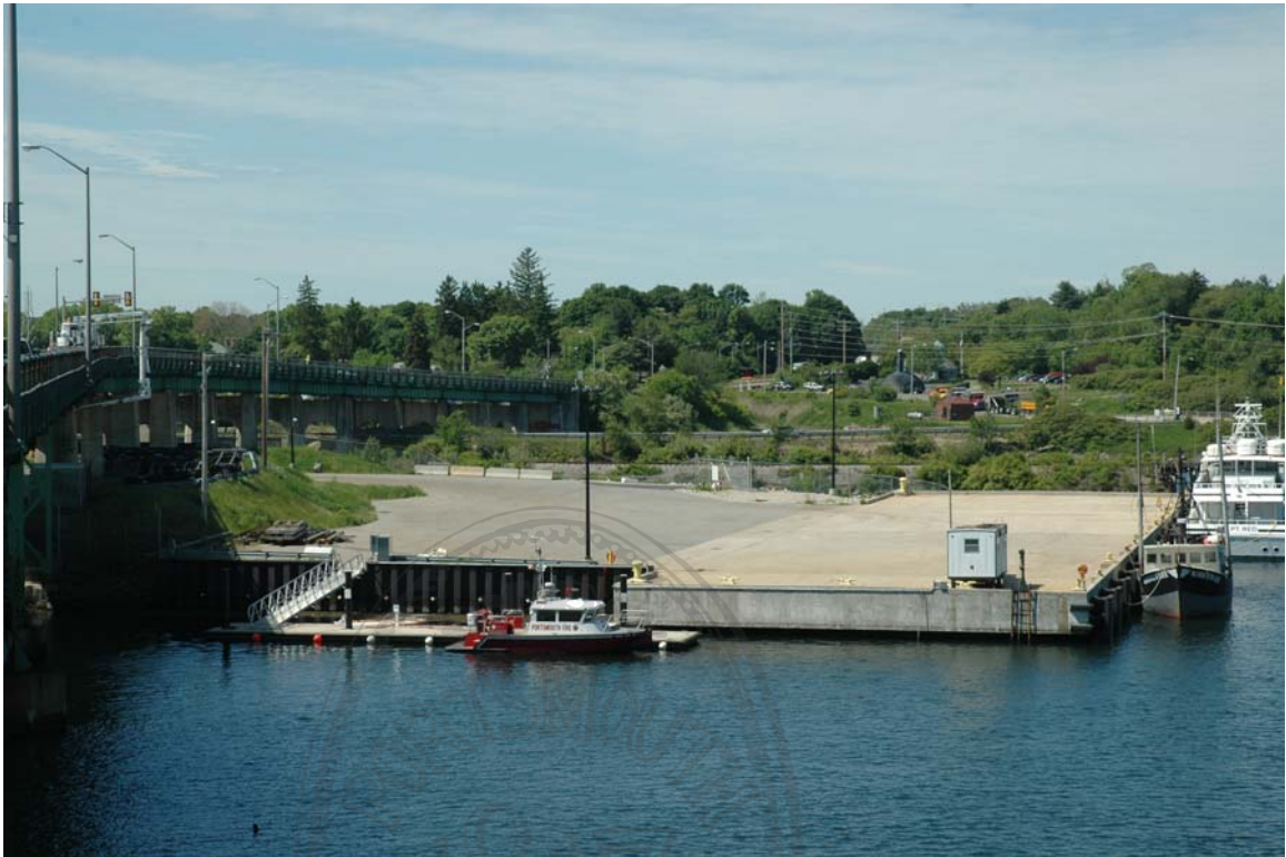
Photo 36) Route 1 Bypass/Sarah Mildred Long Bridge approach and concrete barge Direction: S Digital File: ME-NH_0036
