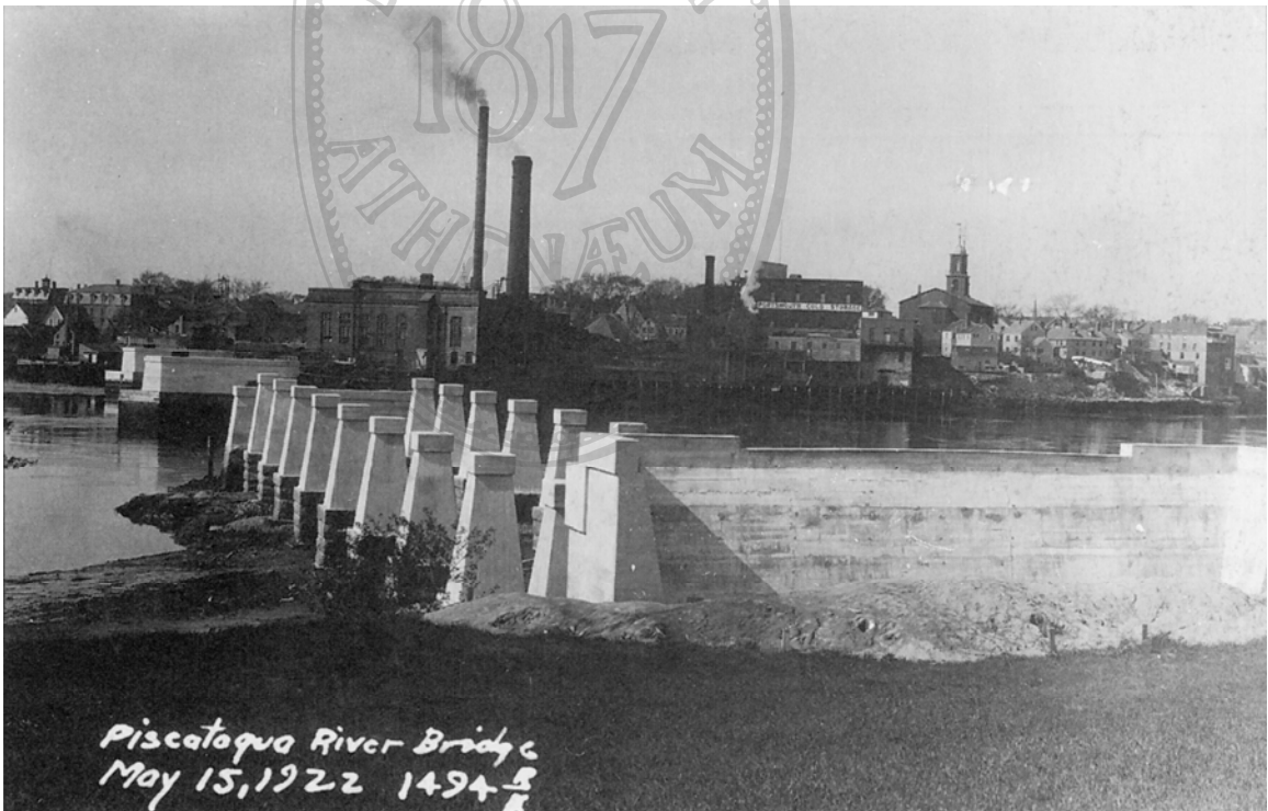
Historic Photo 75) 15 May 1922, looking south from Badger's Island showing concrete shore abutments for Memorial Bridge (Bardwell 1995:45b).
