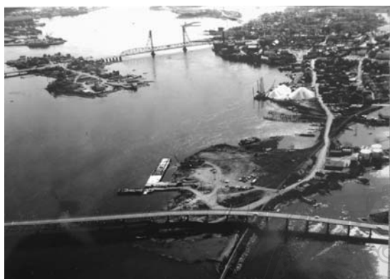
Memorial Bridge and approach to Sarah Mildred Long Bridge
