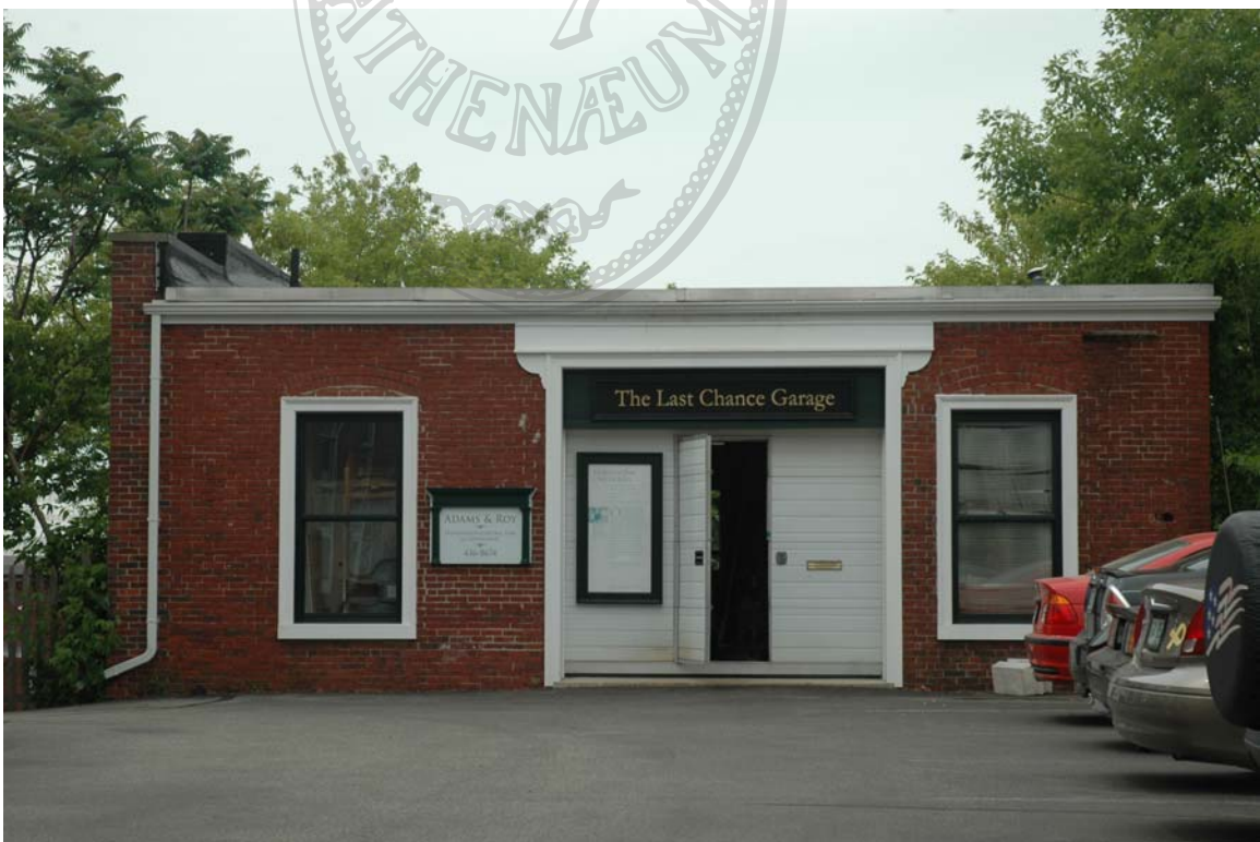
Photo 52) Hill Street, northwest side Direction: NW Digital File: ME-NH_0052
