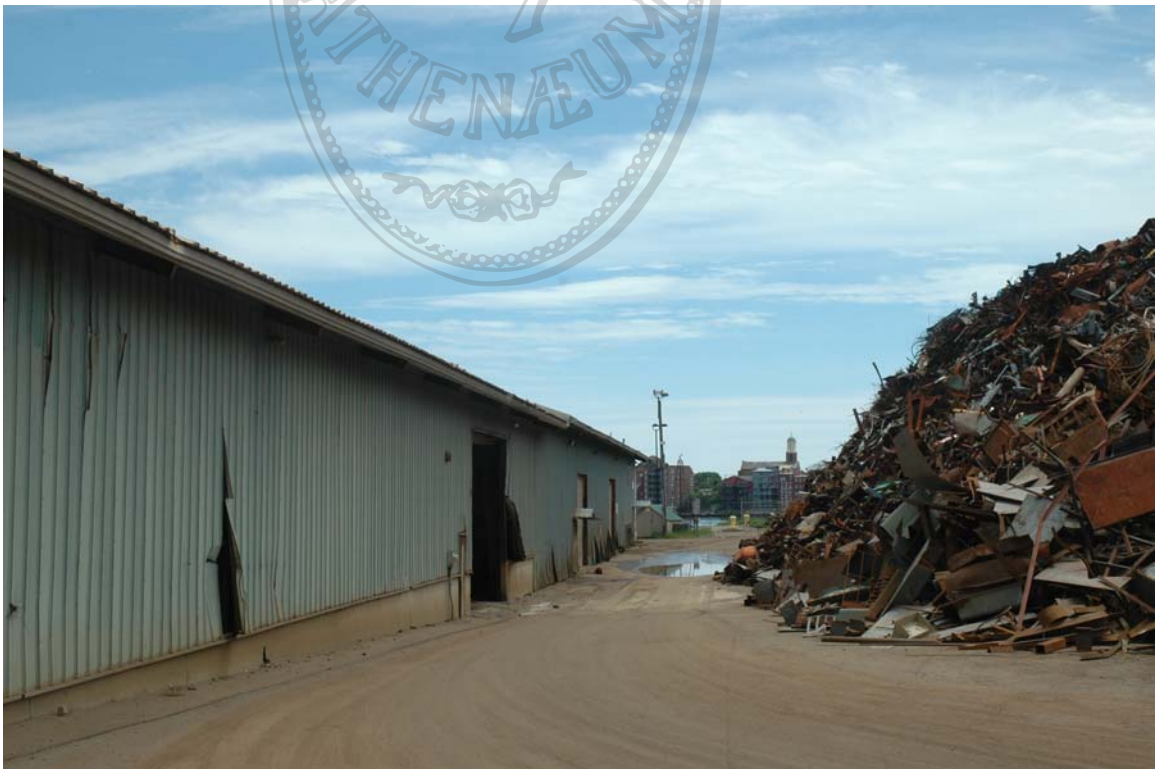
Photo 33) Port building, southwest elevation and scrap pile Direction: SE Digital File: ME-NH_0033
