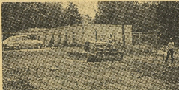
Joe Killeen, treasurer, on bulldozer; Ernie Messier, V.P., at the transit.
