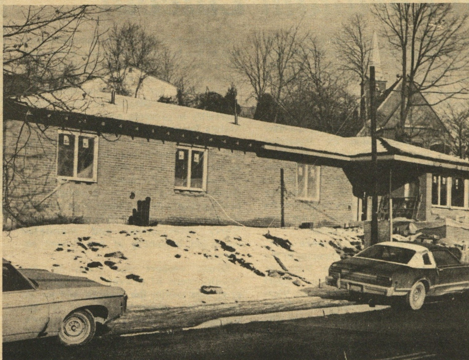
The ULSTER Association for Retarded Children's new Intermediate Care Facility is nearing completion as the photo taken in January will attest. Located on Murray Street in Kingston, the new facility will serve to meet the medical and therapeutic needs of the residents. It is scheduled to open this year.
