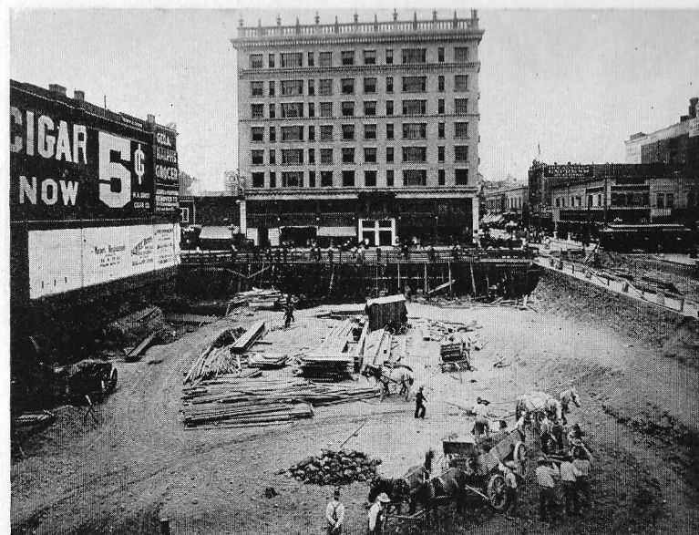
When the excavation was made for the Security Building in 1906 the Alexandria Hotel had just been completed.
