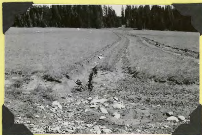
Figure 39. Range access roads on the Bighorn. Erosion control ditching in foreground. These roads are on the maintenance plan and erosion control work is accomplished with road funds. 7/27/55.
