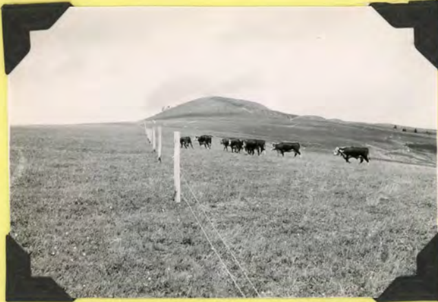
Figure 28. One of the two-wire electric management fences which Ranger Cook uses to good advantage to separate cattle and sheep along high open ridges between allotments. 7/25/55.
