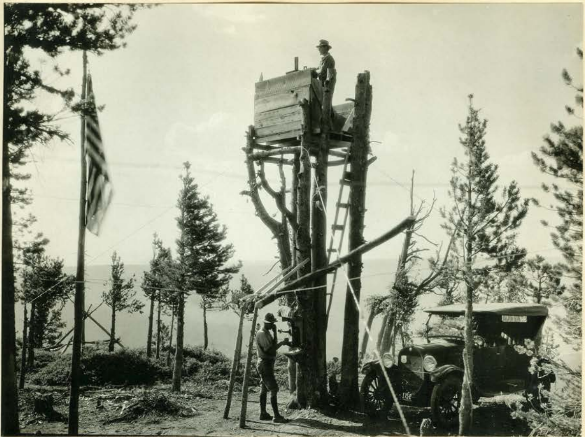
Makeshift arrangement for a lookout tower on one of the lower lookout points on the Fremont N. F. Lookout man exposed to intense sun, wind, and to lightning, which is common in this region. Continuous service in fire detection not Practicable.
