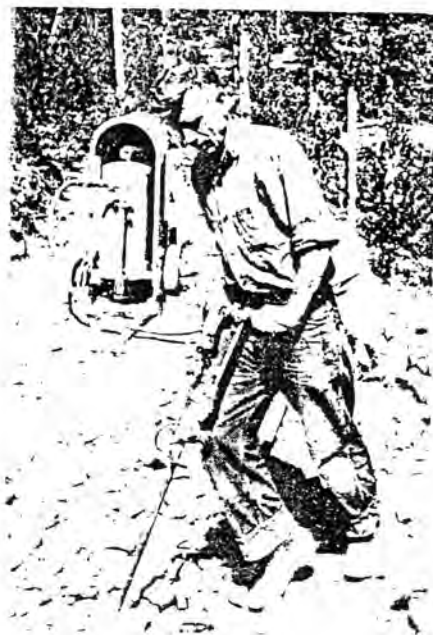
(Above) New model midget truck. Features are overhanging motor suspension, load concentration over rear axle and short turning radius. (Left) Portable air compressor, broken into two parts for field transport, motor on one end, compressor on other. (Below) Breaking rock with portable compressor on forest road job.
