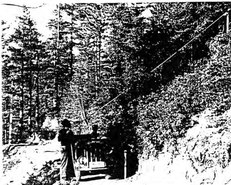
Upper slope stake illustrates actual cross section of excavation and clearing required for standard truck trail road. Compared with narrow excavation required for midget
