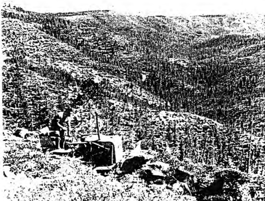
The little tractor can take its share of punishment. Building trail from distant horizons through rock formations. The Japanese incendiary bomb landed near here.
