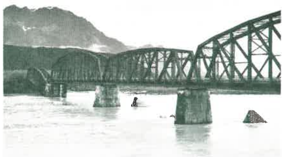
The Million Dollar Bridge near Cordova was constructed in 1909 at a cost of, obviously, $1,000,000. It was heavily damaged in the March 1964 Anchorage earthquake. The bridge spans the Copper River and connects Childs and Miles Glaciers. The damage has had minimal repairs and is used for vehicular travel today.
