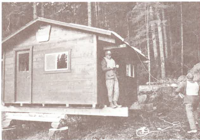
Cabin rests on temporary supports at its new location at Cascade Creek in Thomas Bay. It only took 5 minutes to helicopter the cabin from its Spurt Lake site.
