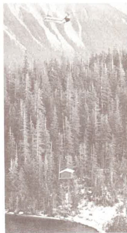
Columbia Helicopter used its Boeing Vertol helicopter to carry the 6,800 pound payload to its new location.
