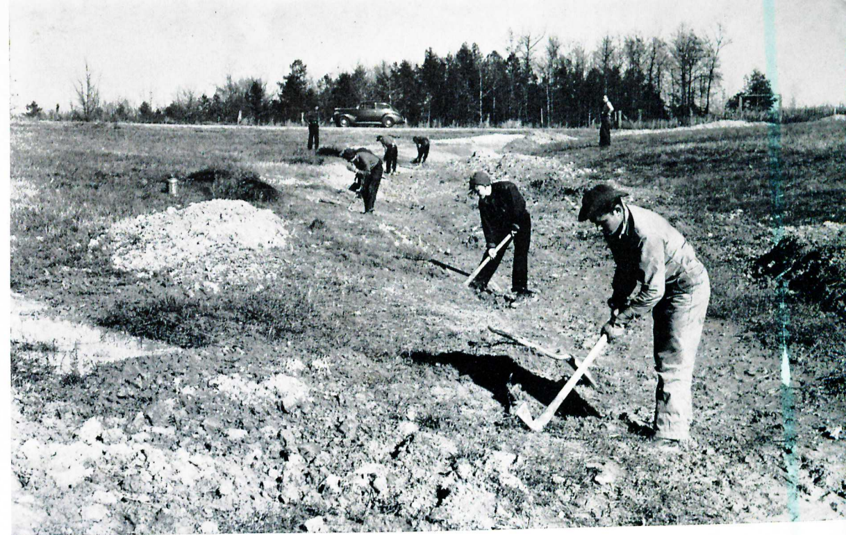
Constructing a Terraced Outlet, one of the enrollee's ways of combatting erosion.
