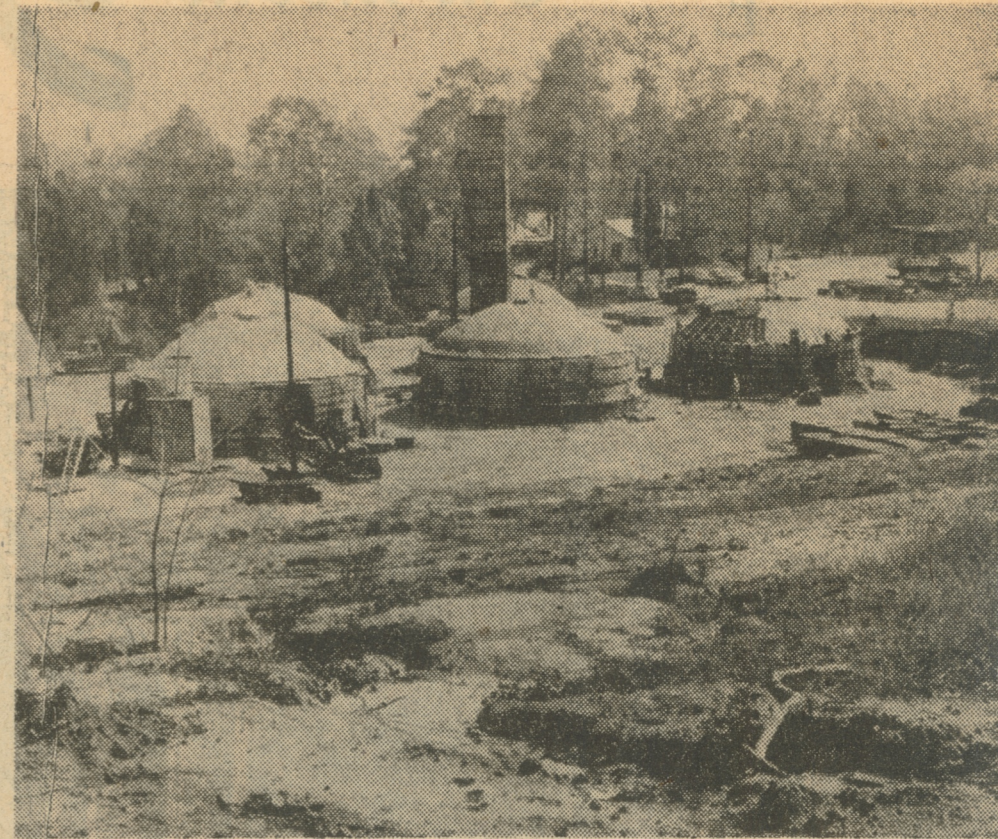
RECEIVING A NEW CROWN —Workmen are busy putting a new crown on one of the five bee-hive type kilns used at the Fairhope brickyard. Automation has taken over most of the operations of the plant and production will be vastly increased.
