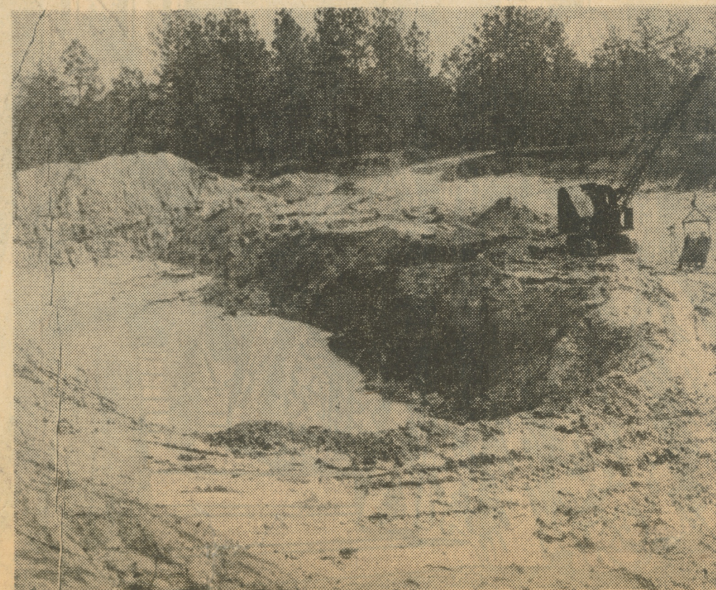
CLAY PIT —This is only one of the many clay pits found in the southeastern section of the state. In the above photo the crane is used to dig the clay from the pit, located near the Fairhope Clay Products Co. The clay is then loaded onto dump trucks to be transported to the brickyard.
