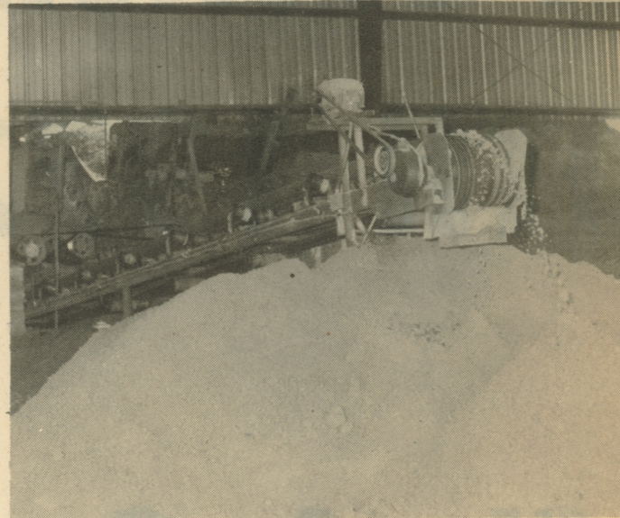
THIS MACHINE grinds, dries, and piles the clay ready to be used. (Photo by Keith Wood)
