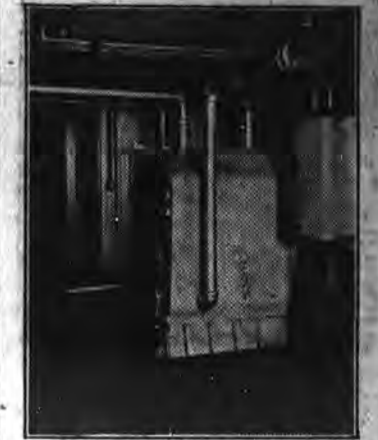
Burner Mechanism Almost Entirely Within Furnace.
