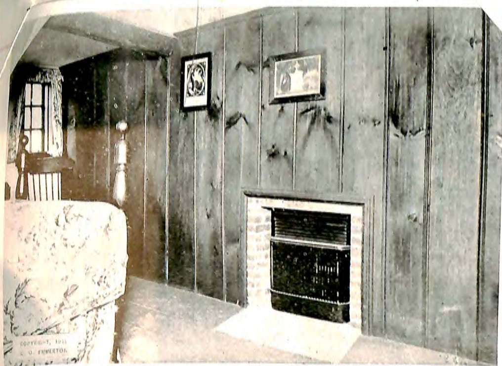
CLIFFORD'S BEDROOM, "THE HOUSE OF THE SEVEN GABLES", Salem, Mass. Showing panel which furnishes entrance to the secret stairway (See panel under star * at top of card)
