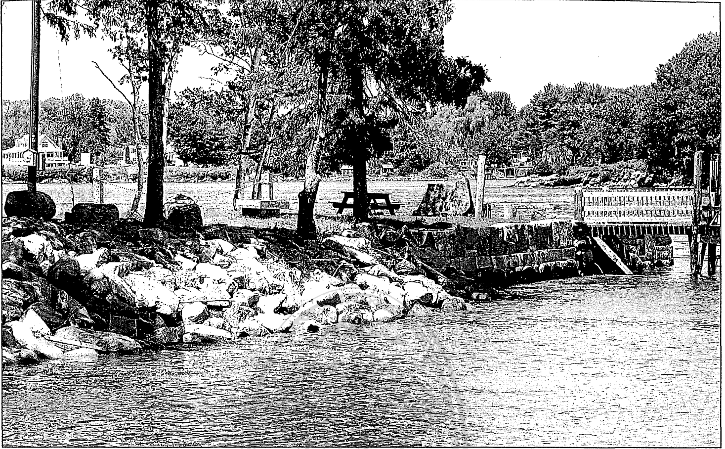
The remains of the Fox Point Bridge abutment showing repairs that were made in 2009 and 2010.
