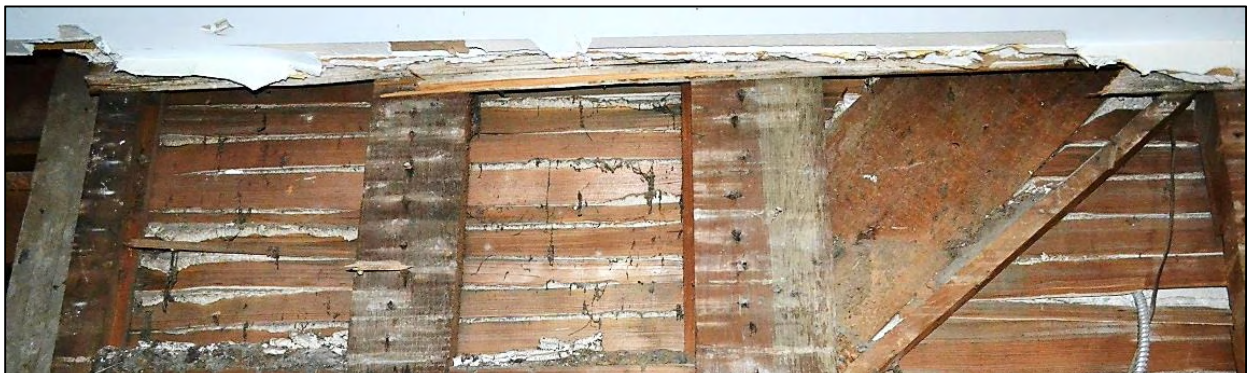
Section of riven (split) pine lath, seen from the southwest front room looking toward the staircase wall and showing the back of the lath strips and the protruding plaster "keys."
