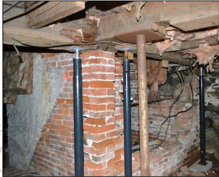
Right: East (side) and north faces of summer kitchen chimney base, showing evidence of former Stairs from the room above.
