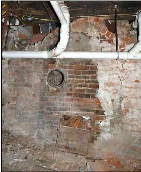
Left: South face of summer kitchen chimney base, showing brick vault (top) and re-used oven door (bottom).
