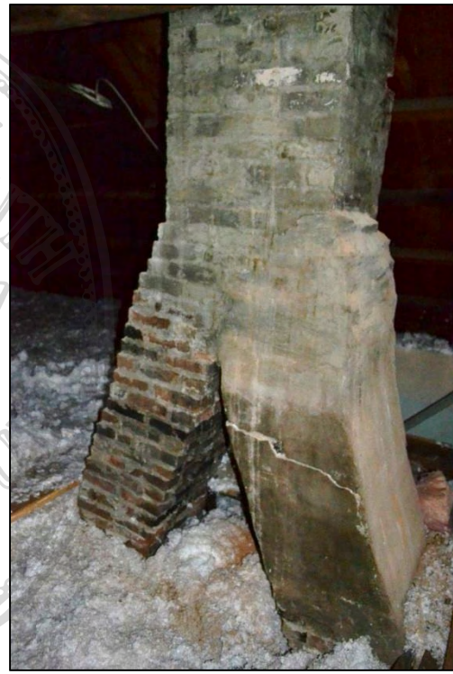
Right: Chimney, camera facing southeast.
