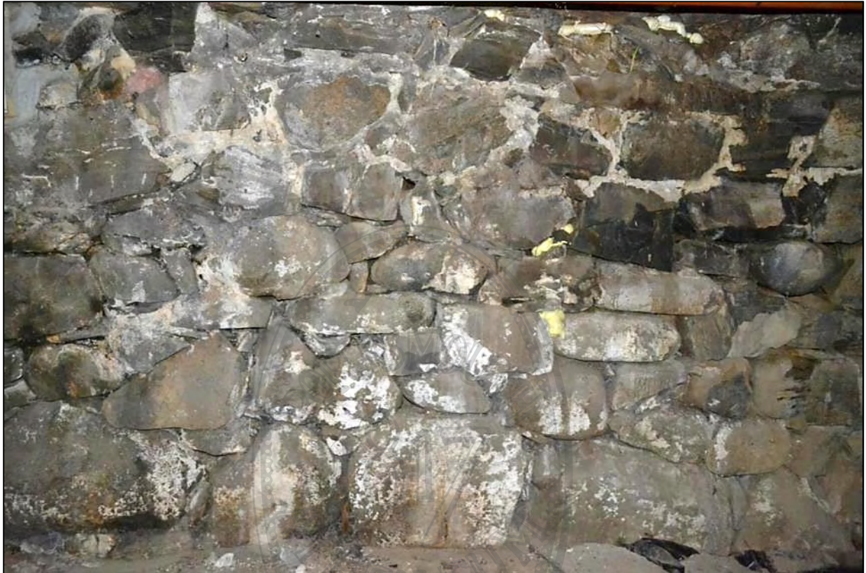
Southern wall of basement, showing natural fieldstones near the base and angular stone near the top. The wall was originally pointed with lime mortar and retains remnants of lime wash (whitewash). The house lacks split granite underpinning at grade level; the mortared angular stone extends above grade to support the house sills.
