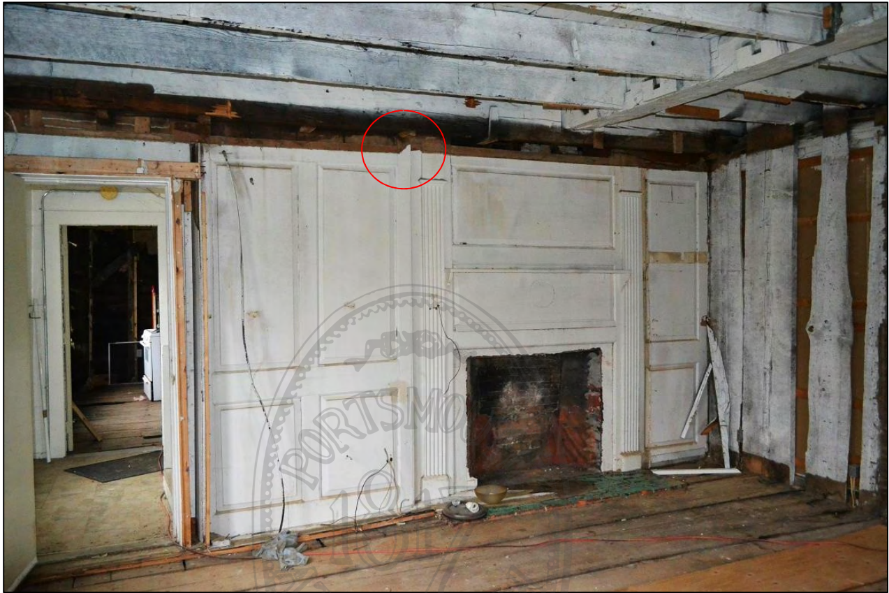
Southeast first-story room (parlor), Dennett House. The panel arrangement and fluted pilasters are common features of Portsmouth houses from the 1750s, but comparable features appeared as early as circa 1730 in the George Jaffrey, Jr., House on Linden Street, off Daniel Street.
