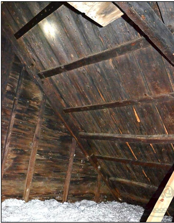
Left: Roof frame, camera facing southeast.
