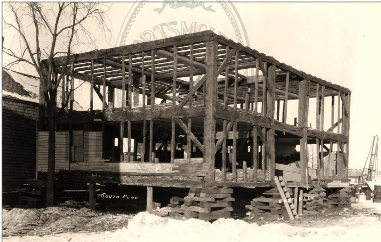
Lieutenant-Governor John Wentworth House (after 1695), shown in 1926 after being moved from its original site and partially disassembled for the sale of its interiors to the Metropolitan Museum of Art, New York. Metropolitan Museum of Art, Sage Fund, 1926. Neg. No. SF 294.
