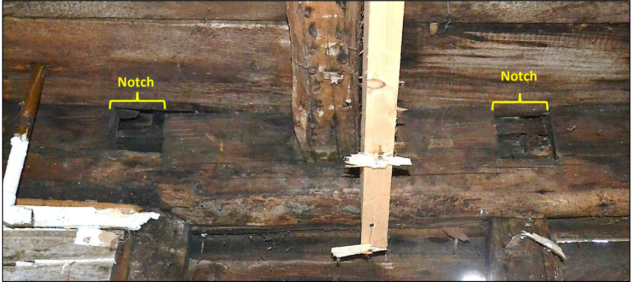
Front girt of Dennett House, southwest first floor room, looking south and showing an original second floor joist (center) and two empty notches for joists (left and right). These details illustrate the use of butt-cogged joist connections and suggest a construction date after 1700.
