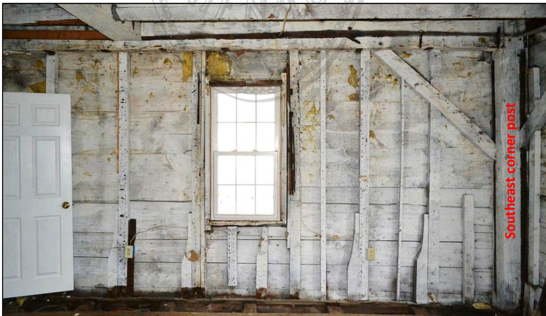
Eastern wall, southeast room. Principal studs may have been sistered during sill repairs.
